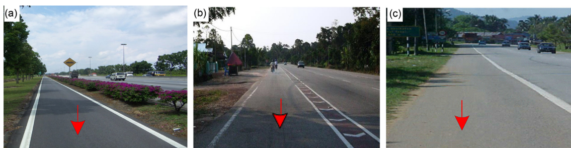
Fig. 2. Illustrations of: (a) an exclusive road lane, (b) an inclusive road lane, and (c) a paved shoulder road lane.
